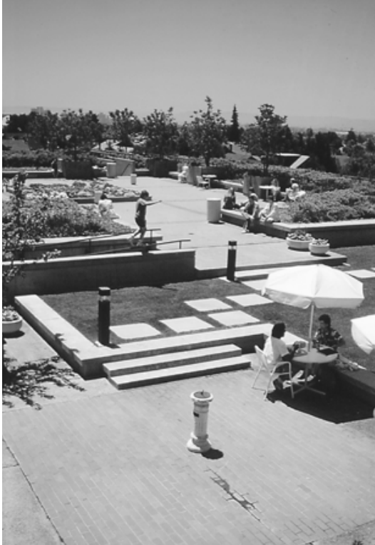
Photo 7-6: The absence of shade and wind protection is apparent in this overview of the roof garden.
