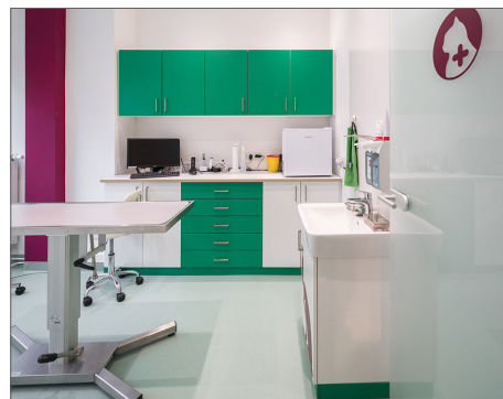
Barenwiese Veterinary Practice: Altro Cantata adhesive-free floor seamlessly integrated with Altro Whiterock wall cladding creating a sealed, watertight system, ideal for areas where safety and hygiene are paramount.
